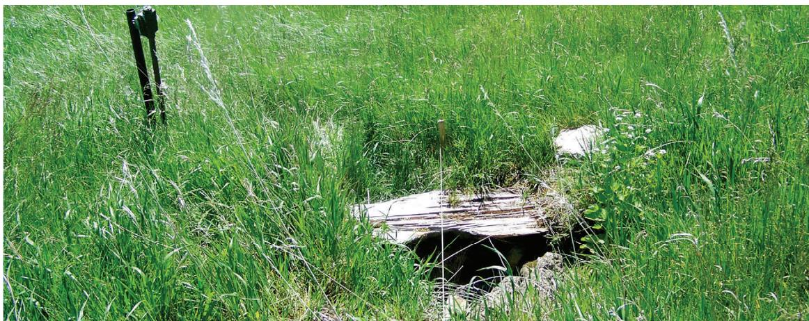
After a summer of digging, the well area now appears as follows. The first effort was to remove the top material, which consisted of long wooden planks, large metal plates and concrete slabs. All of these materials are thought to have been used to cover the well opening for protection from dirt and debris and to allow safe and secure access to remove water from well. The wooden planks were seven feet long and two feet wide with an access hole in the
