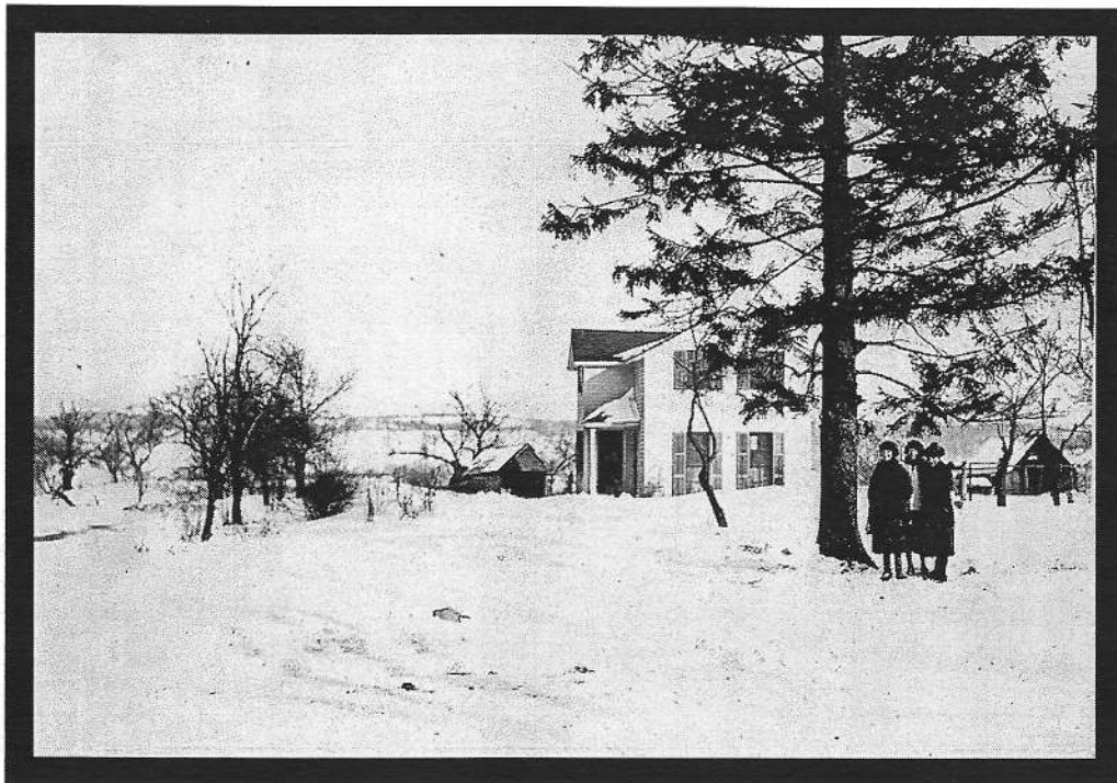
The house at 432 Landing Road, across the street from the Tryon/Pok home, is pictured in winter with a clear view of what is the park today.
