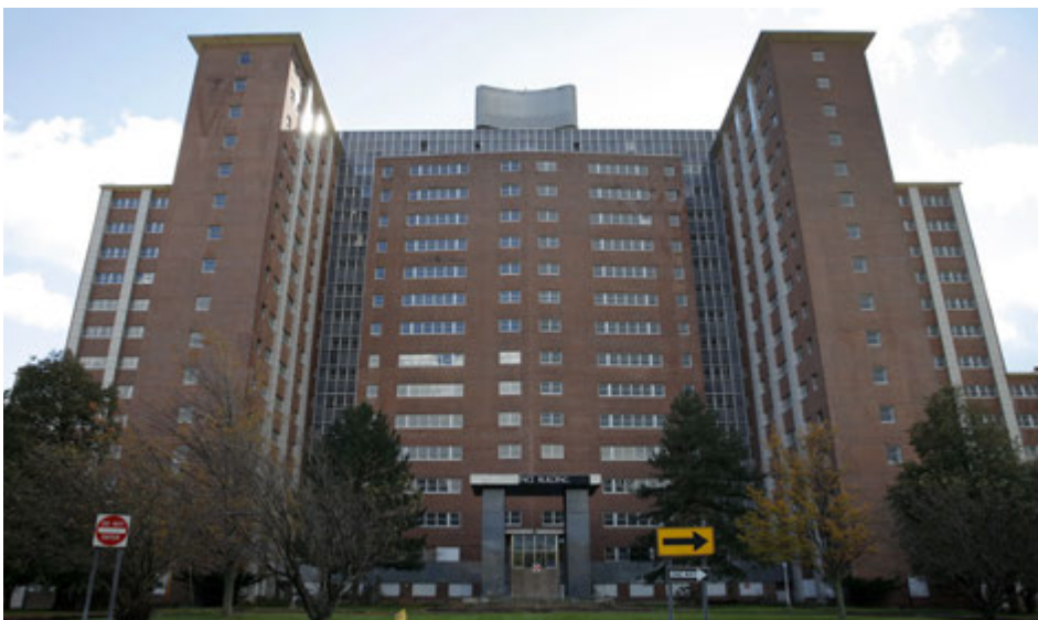
The imposing facade of the Terrence Building looming over Rochester and Brighton, photo from Democrat & Chronicle archives
