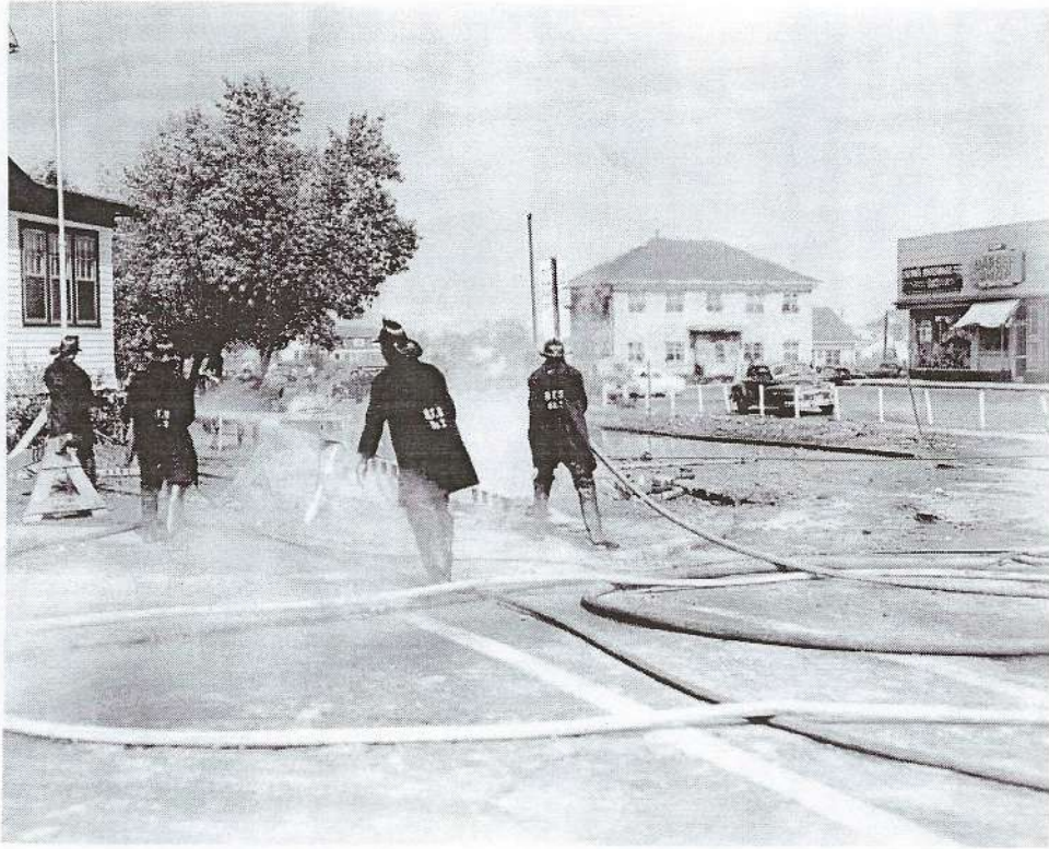
Street view of Monroe Avenue and Winton Road with Brighton firefighters dealing with the fire in the vault. Twelve Corners Plaza on the right.
