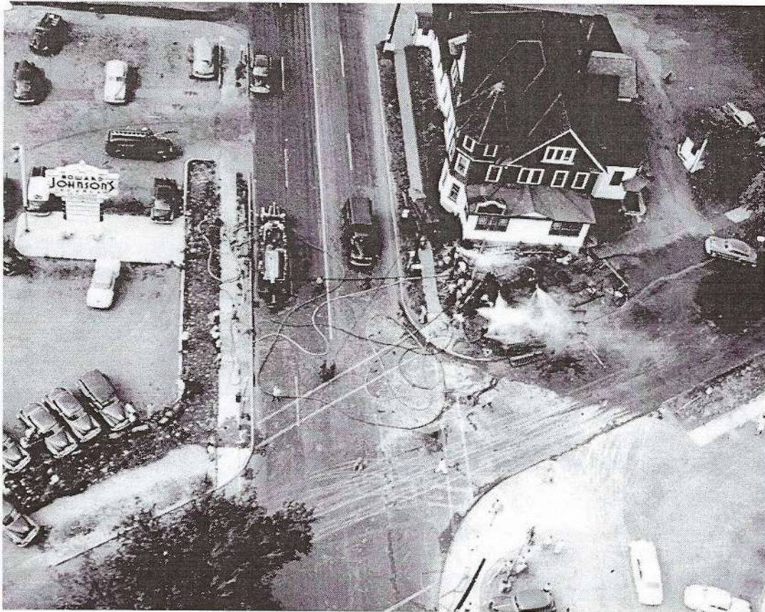
Aerial view of the Monroe Avenue-Winton Road intersection showing Brighton firefighters with hoses and the vault near the Chateau Restaurant.
