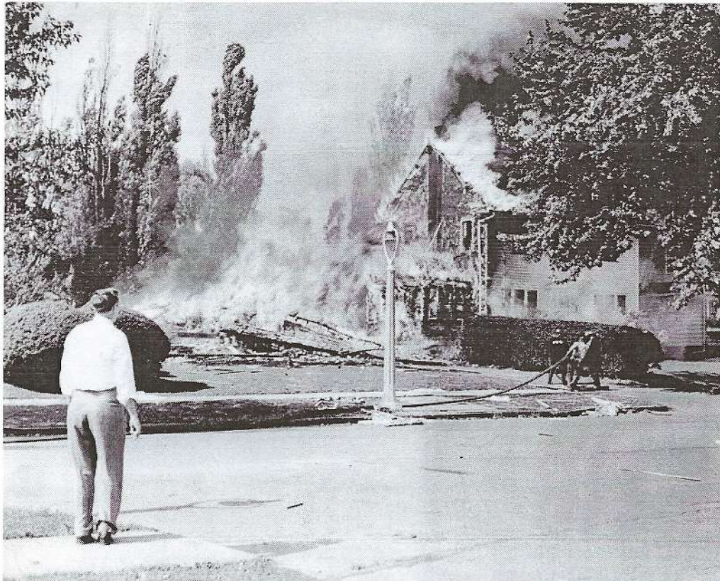
Sylvan Road in Roselawn where one house was destroyed and the house next door badly damaged by fire.
