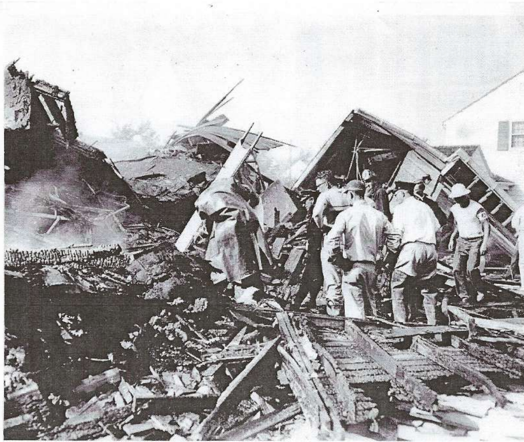
Firefighters, police, and Civil Defense workers at 155 Buckland Avenue in Meadowbrook where Mary Ann and Billy Maas died.
