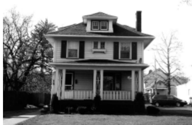
Sylvan Rd.: American Foursquare style with dormers in hipped roof, exquisite wood porch, leaded glass windows and projecting bay on north side.
