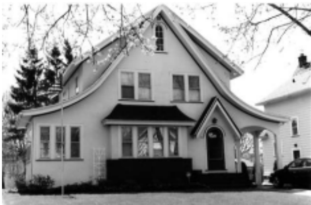
This South St. Regis Drive house is stucco Tudor Revival with porte cochere, steeply pitched roof, and side dormers.
