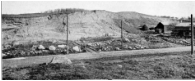
Gideon Cobb's sand bank in the west nose of Cobb's Hill, 1894. The excavation left a wide level area. The hill lost its entire southerly shoulder and huge boulders were dislodged and rolled to the lower ground.
