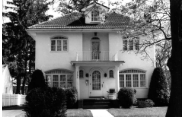
Mediterranean Revival Style on Fair Oaks Ave. White stucco with red terracotta tile roof. Arched transom windows, balcony over the center entrance portico which has Doric columns, and arched entry flanked by two small round-headed windows.
