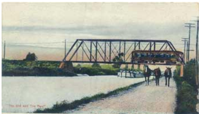
Rail bridge over Erie Canal
